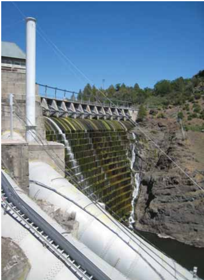
Figure 5-2. Copco 1 Dam showing gated spillway and penstock pipes
