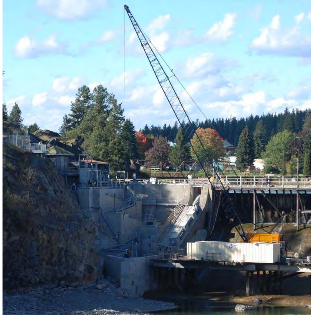
Figure 5-26. Typical Construction Techniques for Building Reinforced, Cast-in-Place Concrete Fish Ladder Using Lattice Crane and Temporary Access Platform at Thompson Falls Dam (photo courtesy of GEI Consultants)
