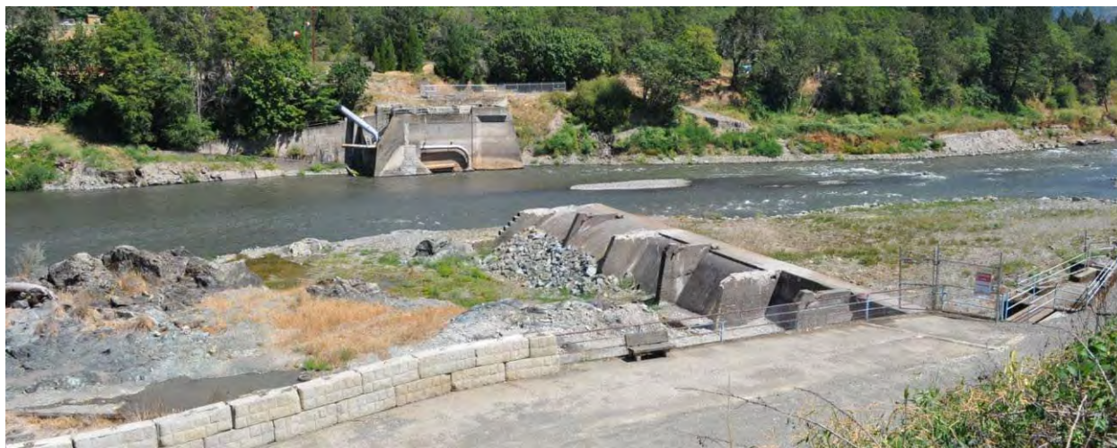
Figure 5-14. Example of Partial Dam removal showing Savage Rapids Dam on the Rogue River (2010)
