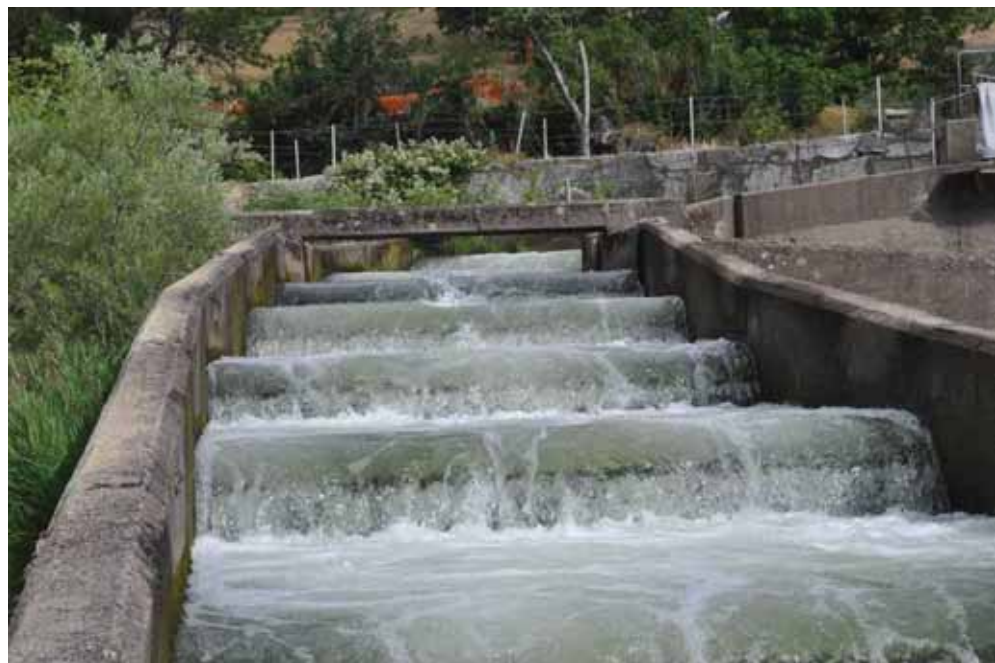
Figure 5-17. Example of Cast-in-Place Pool and Weir Fish Ladder
