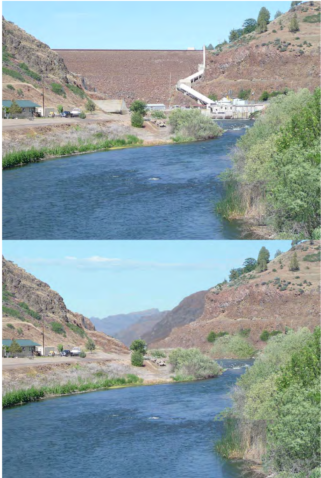
Figure 3-1. Iron Gate Dam before removal (on top) and a simulation of what the facility could look like after full removal (on the bottom)
