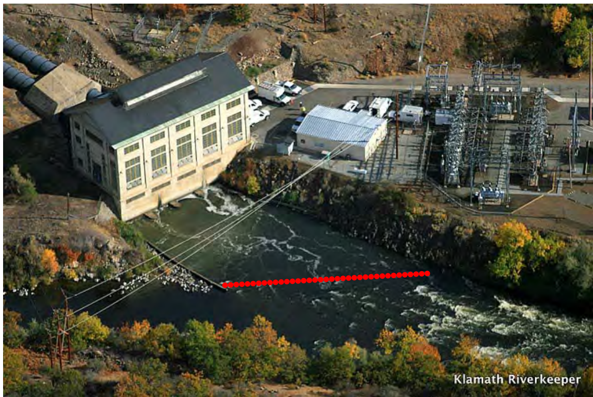
Figure 5-24. Modifications at the Tailrace of the Copco 2 Powerplant would extend the bank and install a tailrace barrier screen (red dots) (photo from Klamath Riverkeeper)
