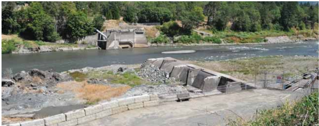
Figure 5-14. Example of Partial Dam removal showing Savage Rapids Dam on the Rogue River (2010)
