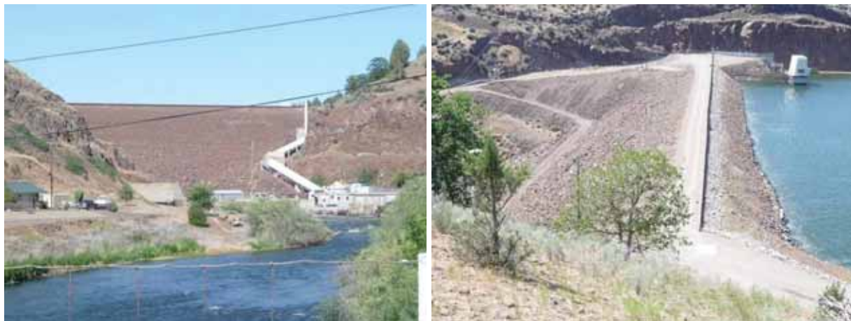
Figure 5-4. Iron Gate Dam (left photo) power generating facilities (left photo) and dam crest and parapet sheet pile wall (right photo)
