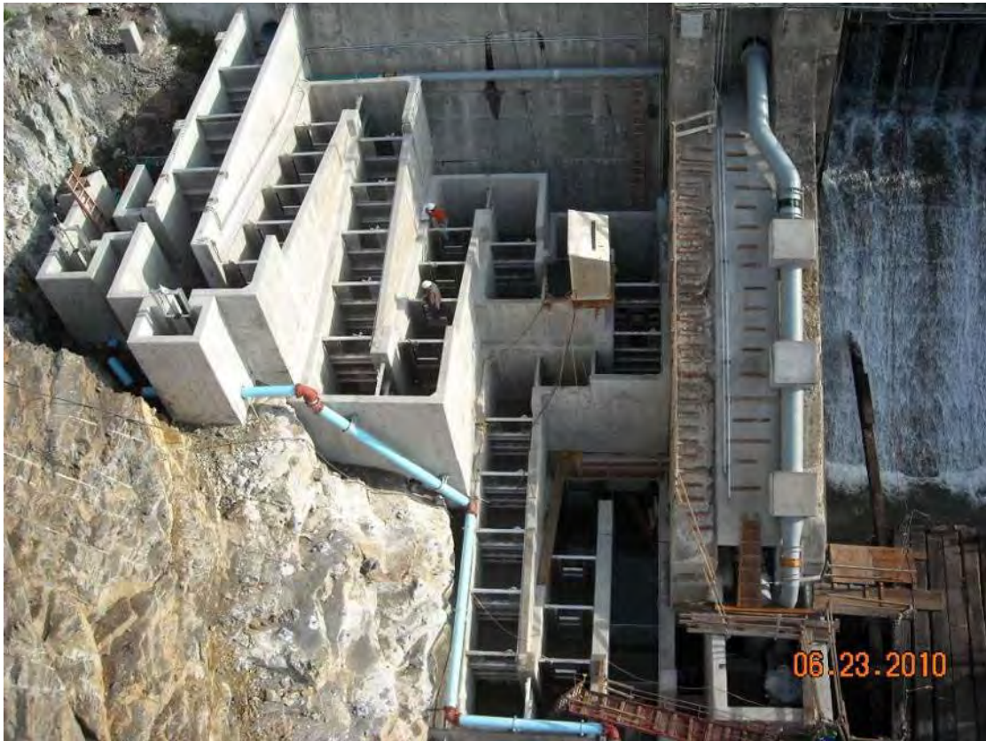
Figure 5-21. Example of Fish Ladder Built into Steep Bedrock Similar to Copco 1 Option (photo courtesy of GEI Consultants)
