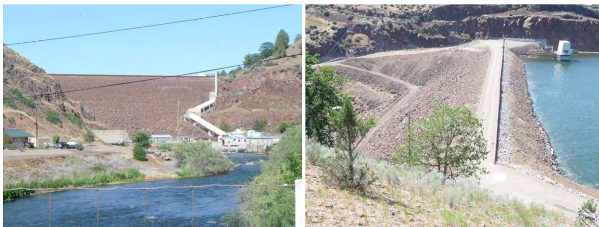
Figure 5-4. Iron Gate Dam (left photo) power generating facilities (left photo) and dam crest and parapet sheet pile wall (right photo)
