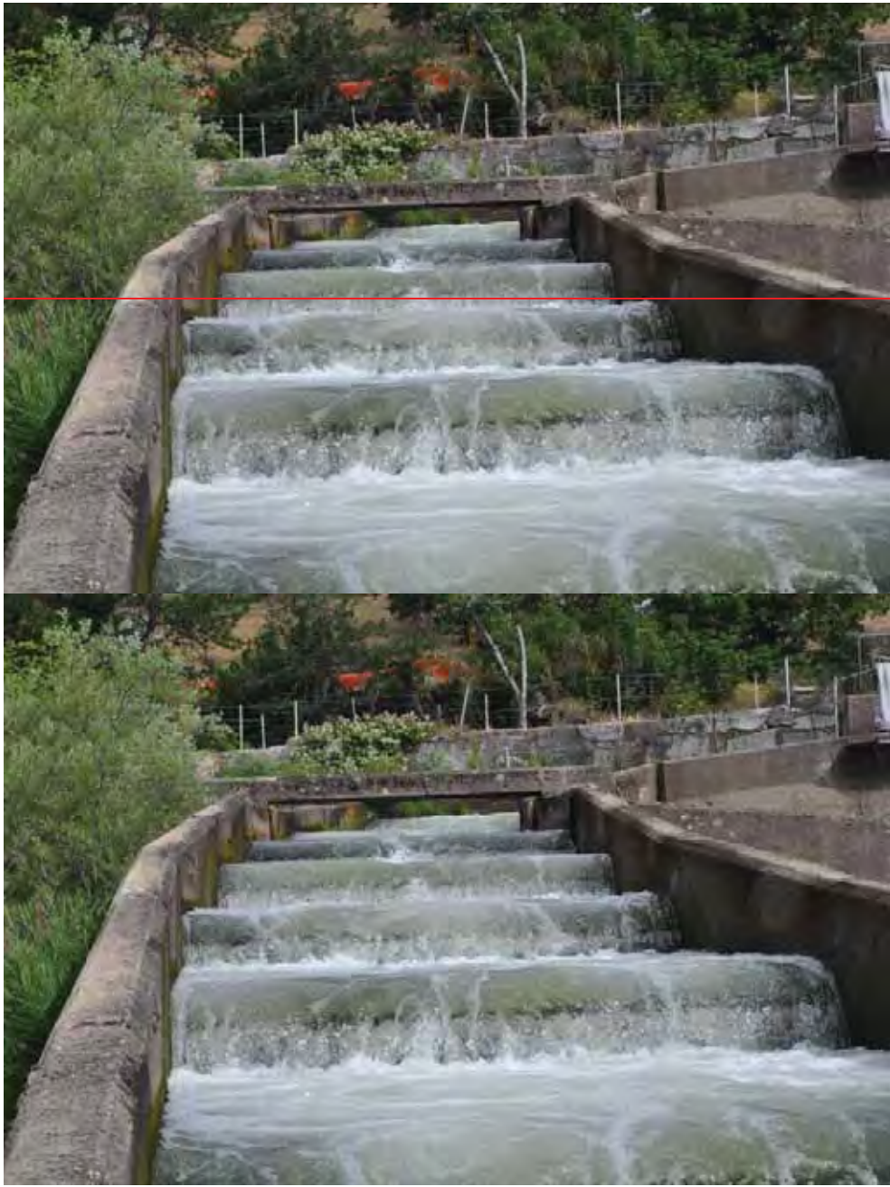
Figure 2-22. Example of cast-in-place pool and weir fish ladder.
