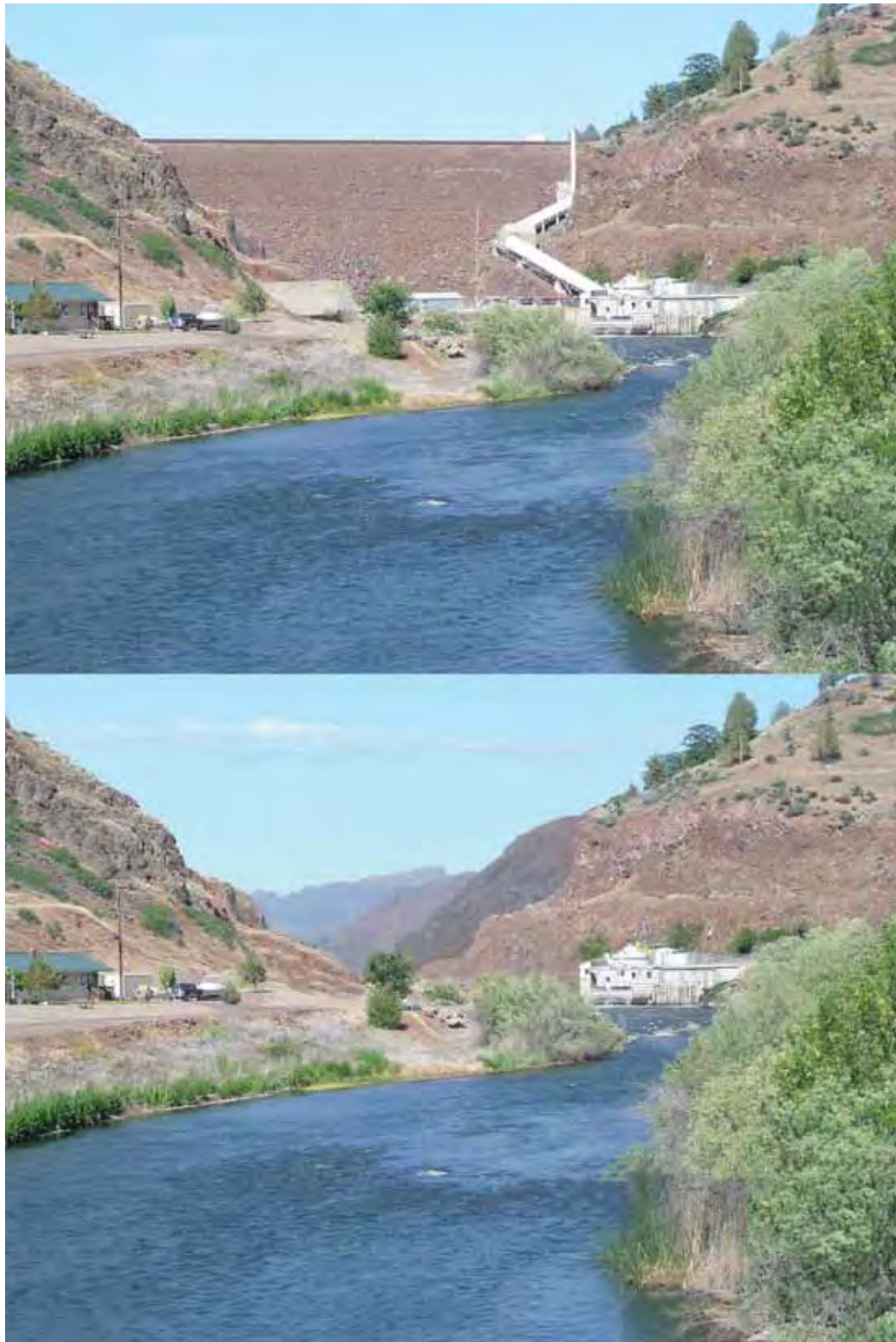
Figure 3-5. Iron Gate Dam before deconstruction (on top) and a simulation of what the facility could look like after partial facilities removal (on the bottom)
