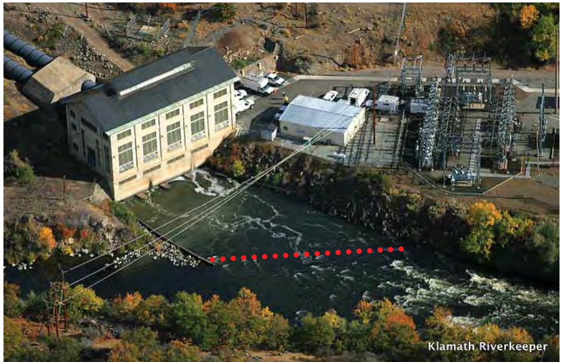
Figure 2-27. Modifications at the tailrace of the Copco-2 Powerplant would extend the bank and install a tailrace barrier screen (red dots) (Source: Klamath Riverkeeper)
