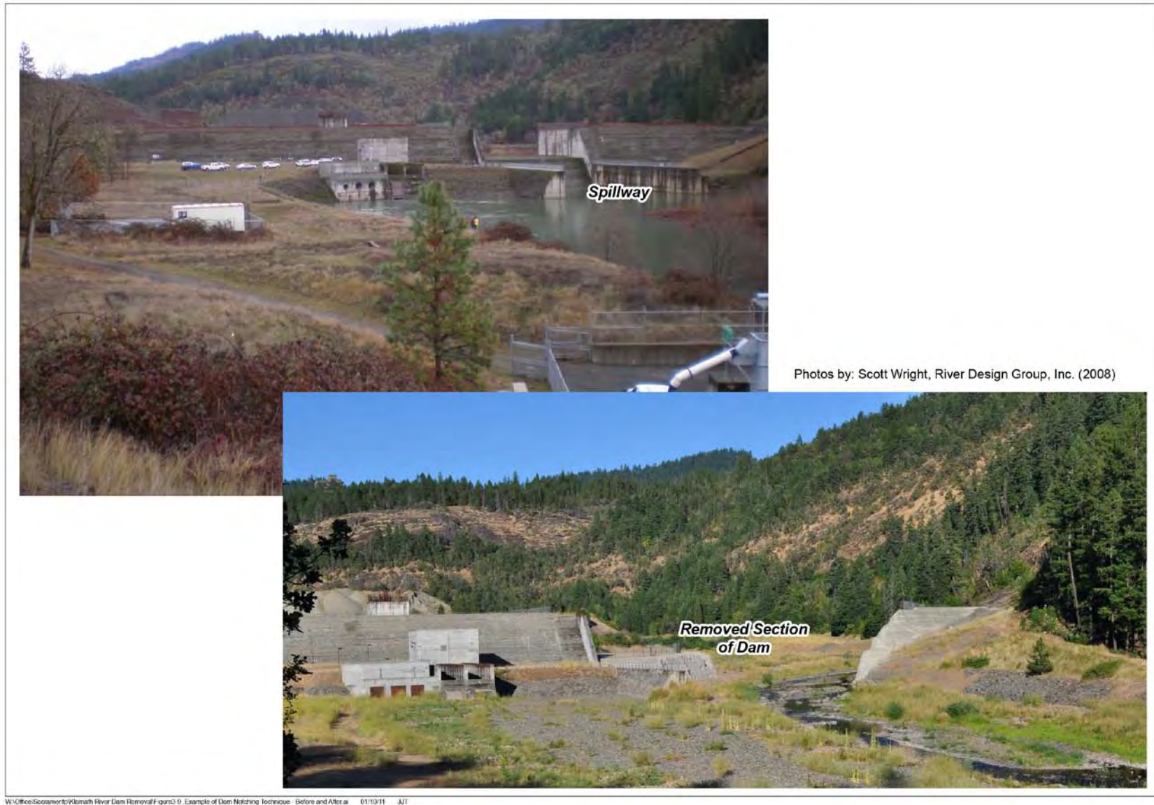
Figure 3-9. Example of Dam Notching Technique, Before and After
