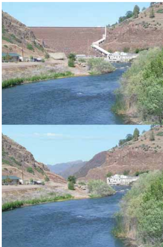
Figure ES-9. Simulation of Partial Facilities Removal
