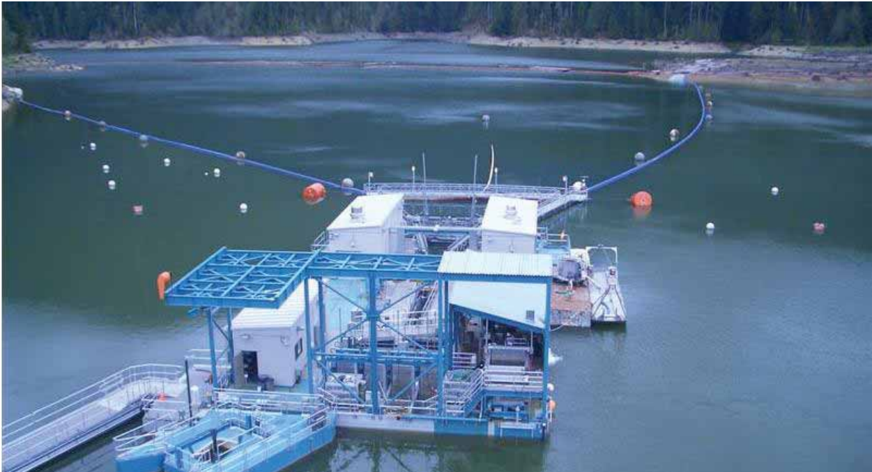
Figure 5-22. Example of Floating Surface Bypass Collector in Upper Baker Dam, Washington (photo courtesy of NOAA Fisheries Service)
